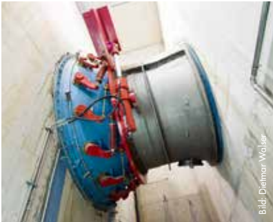
Kaplan-Bulb-Turbine
